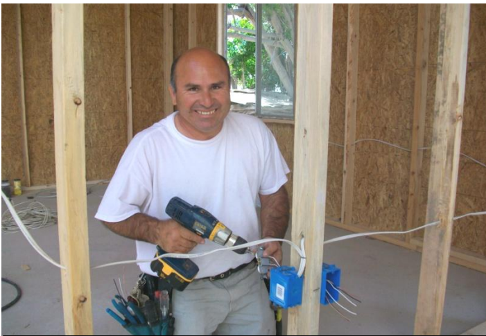
Enrique (PCF) installs electrical wiring.
