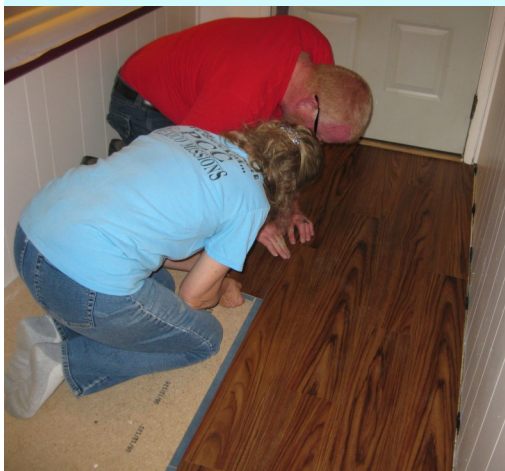
Sam and Jan install “plank” flooring in entryway
